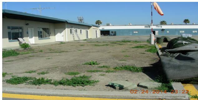
Work in progress on the turf project
